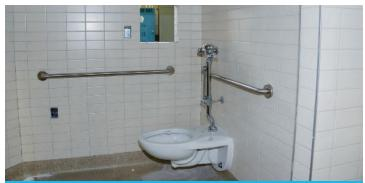
The finished bathroom pods arrive at the job site with toilet, sink and other fixtures in place and ready to use once the final piping connections are made.
